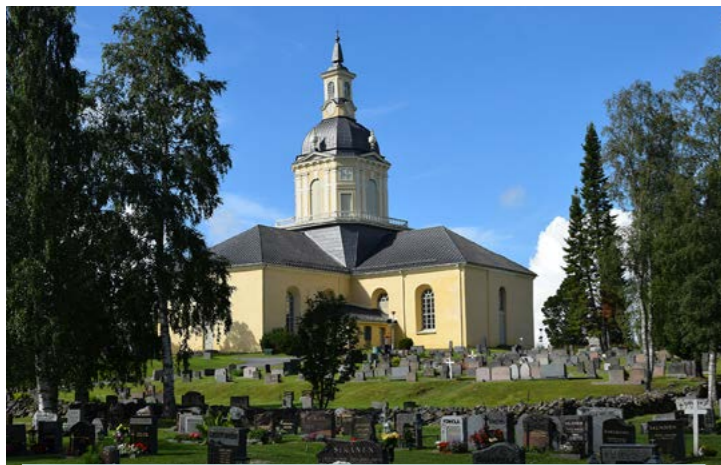
The Alatornio church is located on the Pirkkiö island, where measurements were taken by scientists from Pulkovo, Russia and Sweden. Photo: Jarno Niskala.
